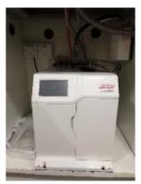
The cupboard the under-counter heating/chilling unit is currently in is: width: 56cm / height: 56cm / deep: 50cm. The unit itself is width: 28cm / hight 33cm / depth 46cm.
