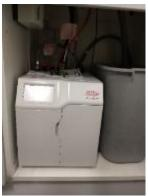
The heating unit for this tap is width: 28cm / depth 31.5cm / height 33cm.
